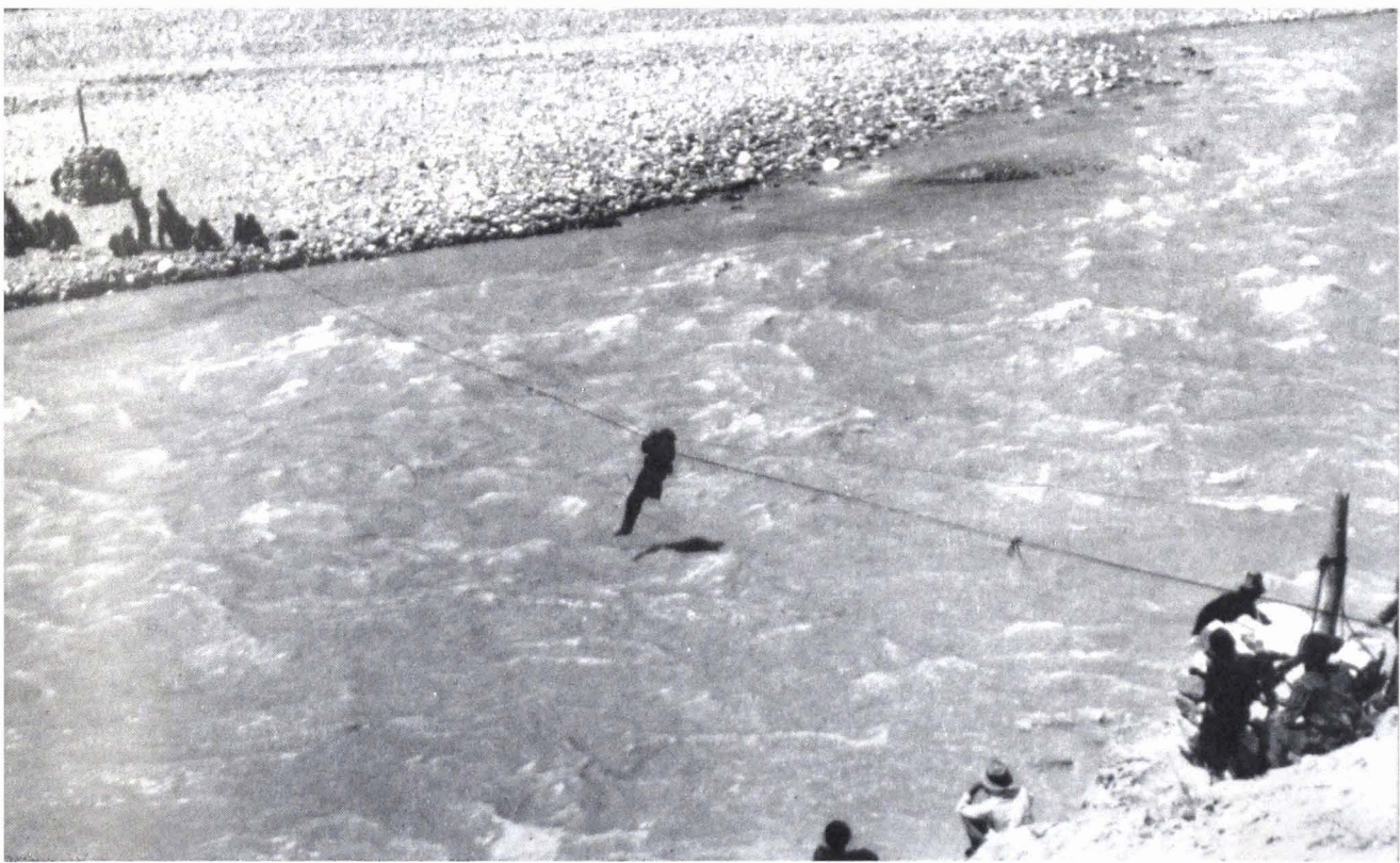
Rope bridge across the Pin river. The passenger is suspended from a rope or cable stretched across the river and pulled across
